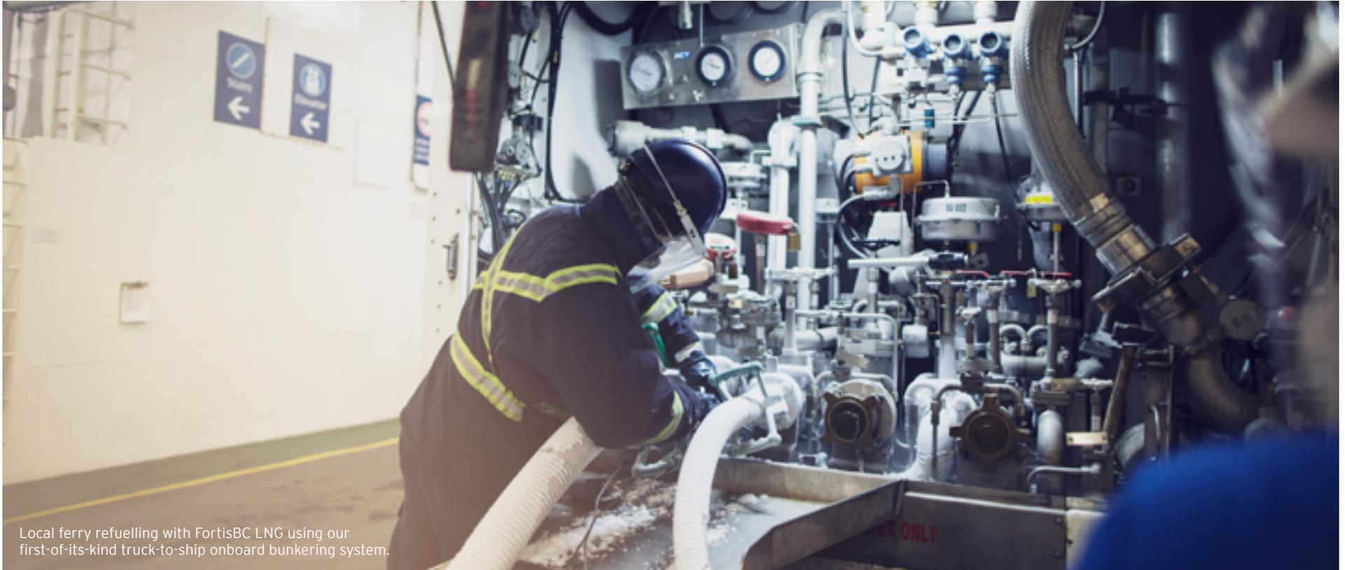
Local ferry refuelling with FortisBC LNG using our first-of-its-kind truck-to-ship onboard bunkering system.
