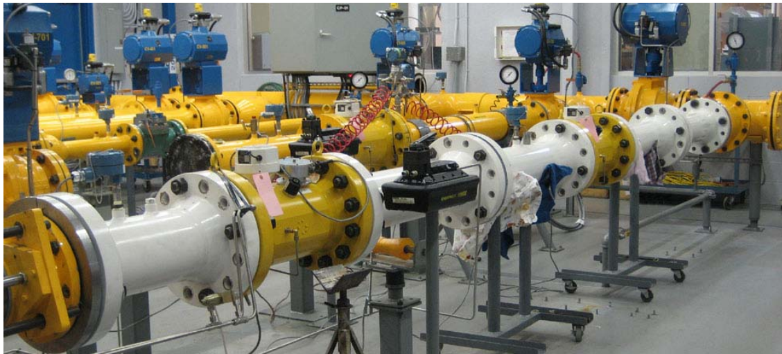
“WATCHDOG” artifact being tested at the Triple Point facility - 2014
