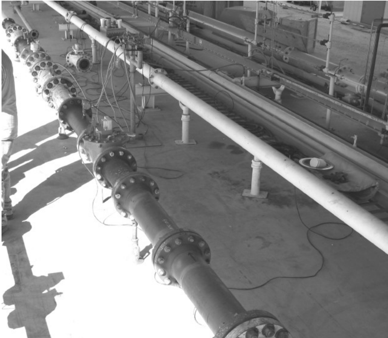
MRF Low Pressure Loop Installation of 8-inch Turbine Meters – Looking Downstream
