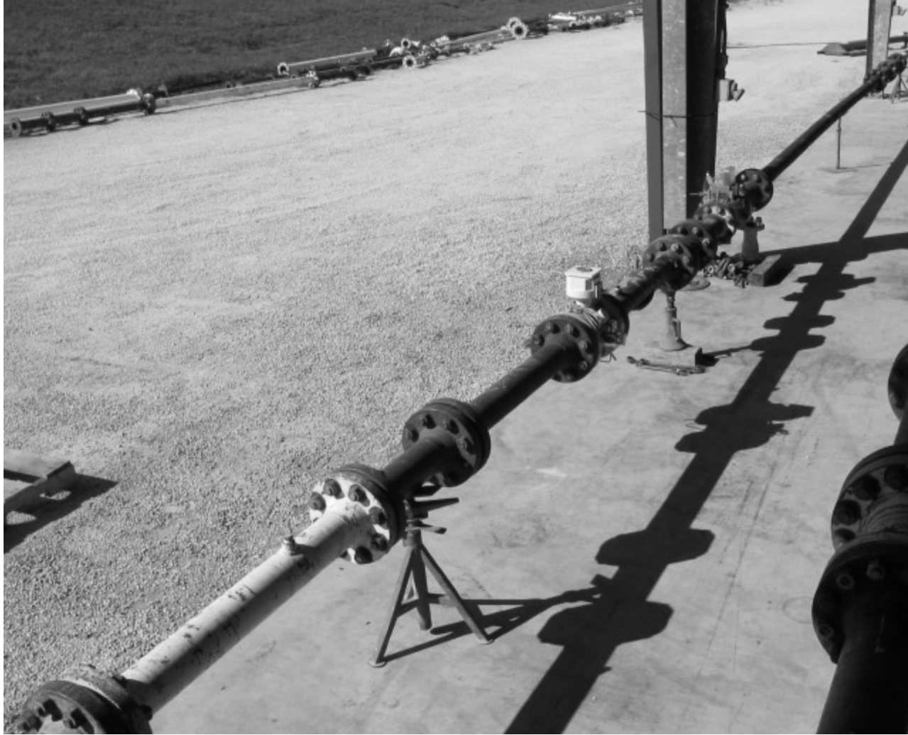
MRF Low Pressure Loop Installation of 4-inch Turbine Meters – Looking Downstream
