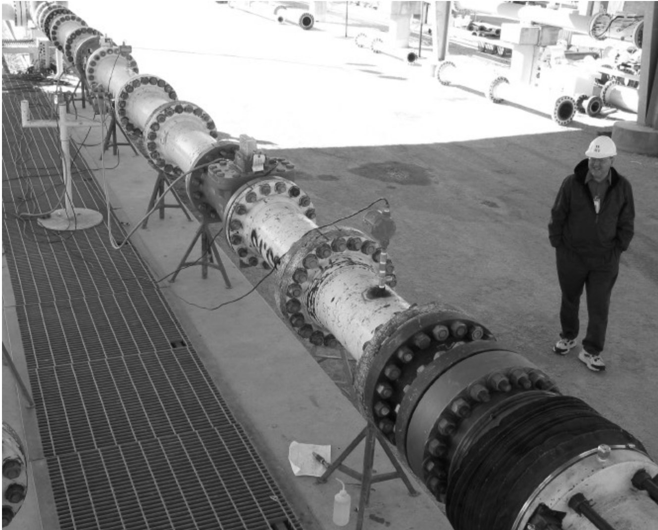
MRF High Pressure Loop Installation of 12-inch Turbine Meters – Looking Upstream
