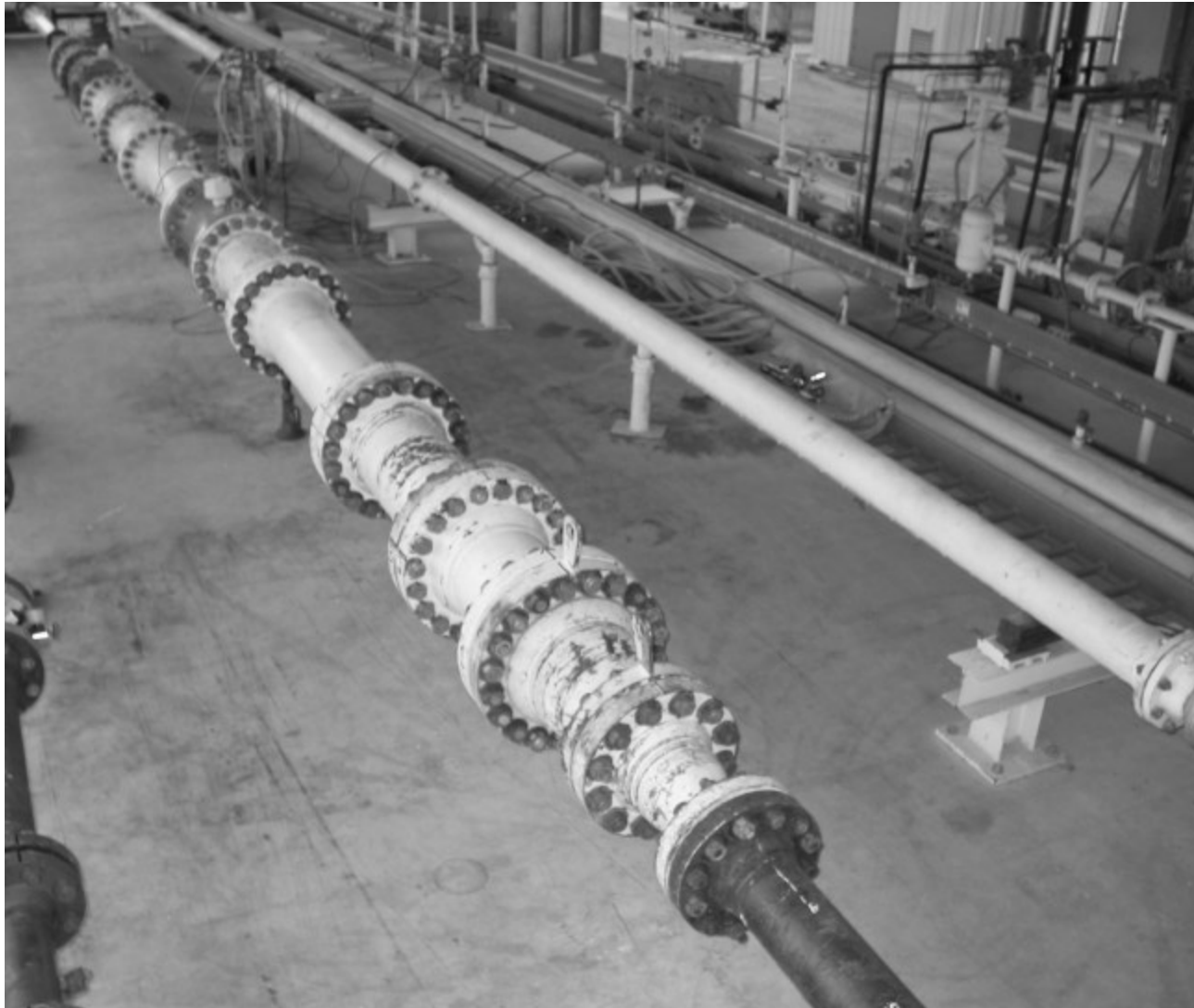
MRF Low Pressure Loop Installation of 12-inch Turbine Meters – Looking Downstream
