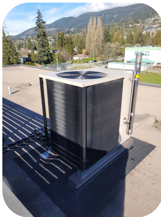
Figure 3: Single GAHP unit installation in BC's lower mainland.
