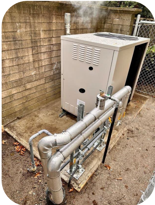
Figure 21: GAHP in operation to support domestic hot water load in the BC's lower mainland.
