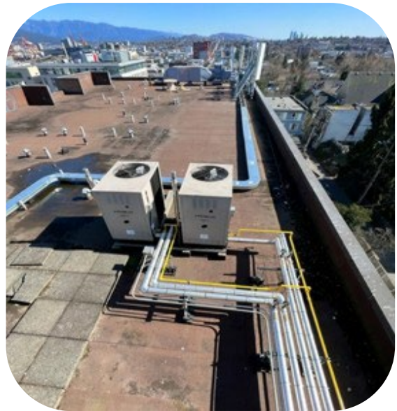
Figure 19: Rooftop installation of GAHPs in Vancouver, BC.
