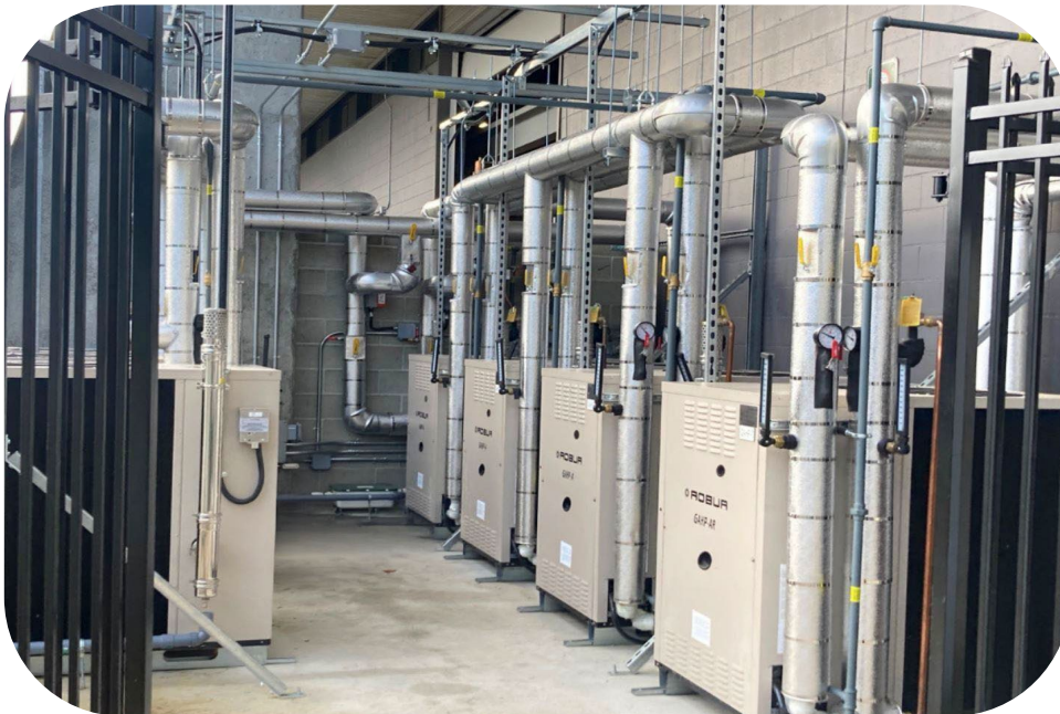
Figure 20: Multi-unit GAHP installation at a project site in Chilliwack, BC.
