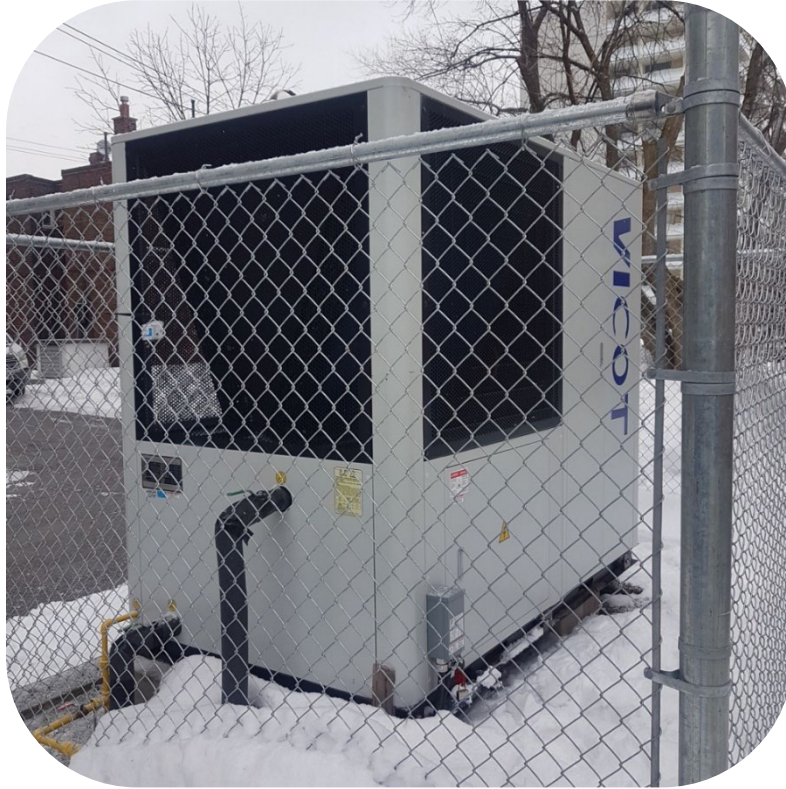
Figure 22: A GAHP unit installed in Ontario.
