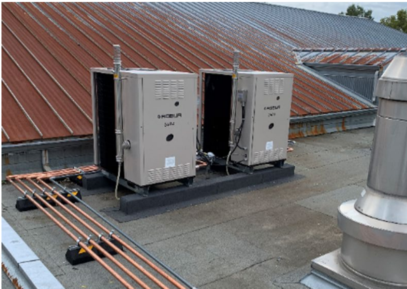
Figure 8: Left: Robur units installed on a rooftop. Right: Pump skid with a buffer tank and glycol feeder.
