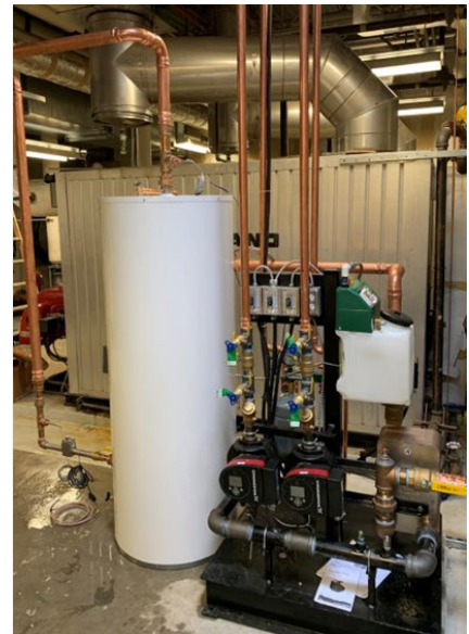
Figure 8: Left: Robur units installed on a rooftop. Right: Pump skid with a buffer tank and glycol feeder.
