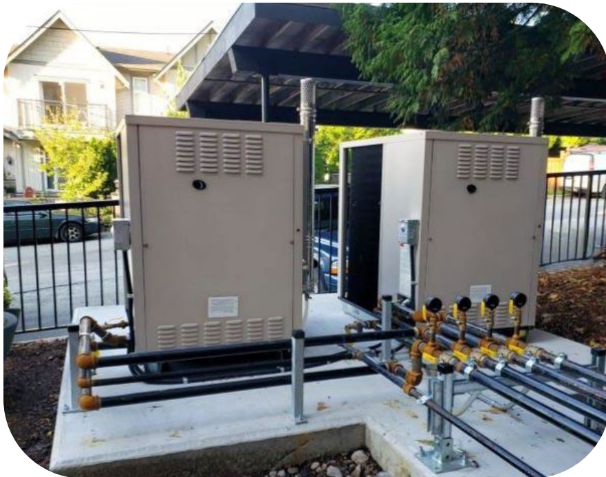
Figure 7: GAHP units installed in BC's lower mainland during FortisBC's pilot stage.
