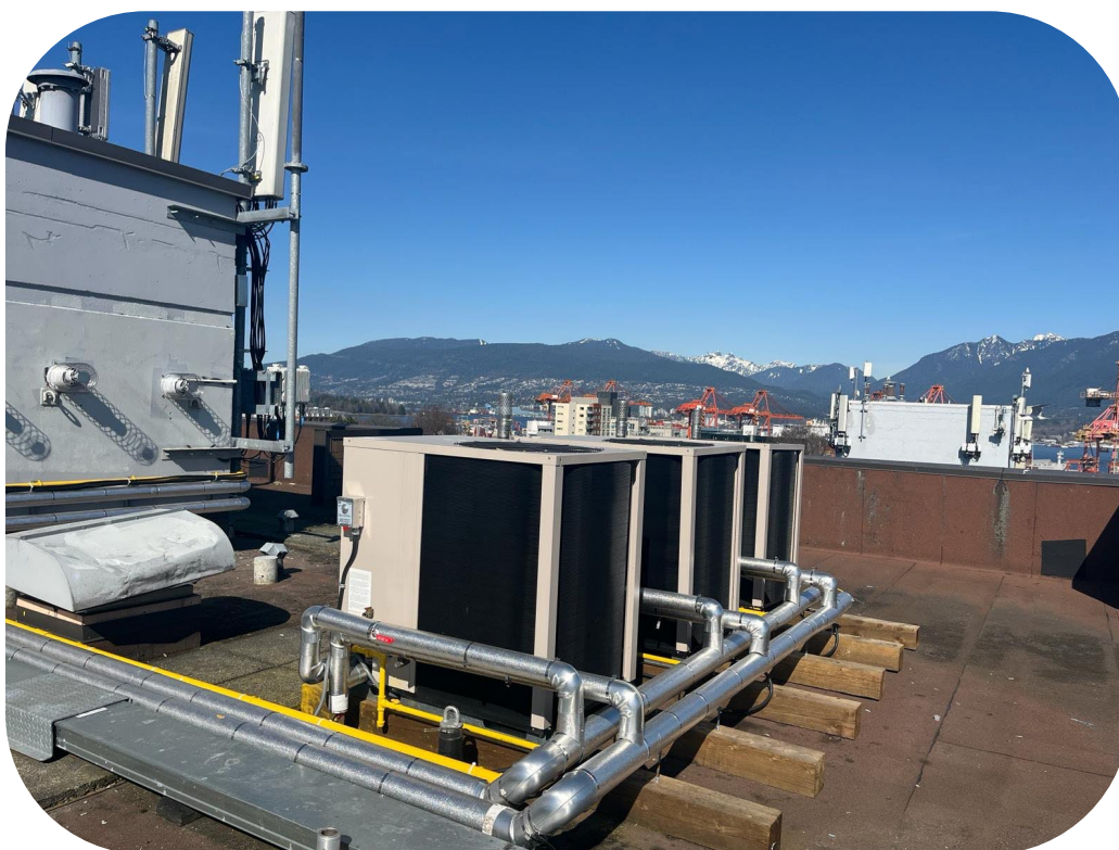
Figure 2: GAHP units in operation in BC's lower mainland.
