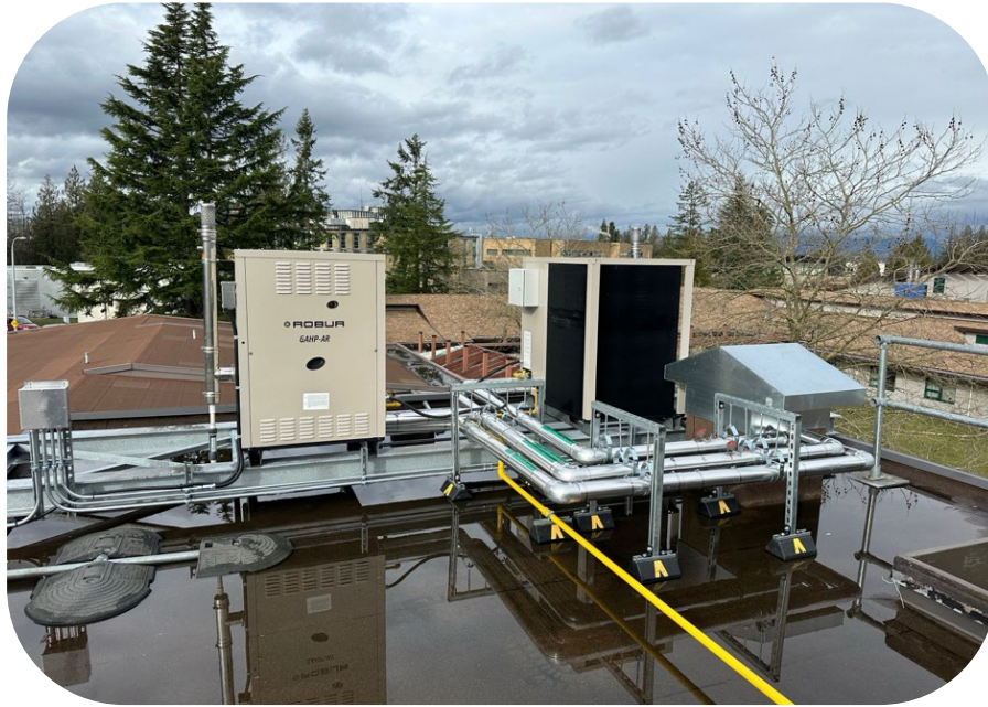
Figure 13: GAHP-AR units installed on a rooftop for a space heating and supplementary cooling pilot in BC's lower mainland.
