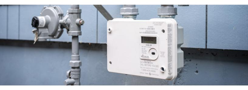
Gas meter exchanges are underway across B.C. as part of FortisBC's Gas Advanced Metering Infrastructure Project. More than one million FortisBC gas customers will have their meters upgraded to wireless advanced meters over the next few years. Increasingly, you'll be seeing the new Sonix IQ advanced meters installed at your customers' homes and businesses.
