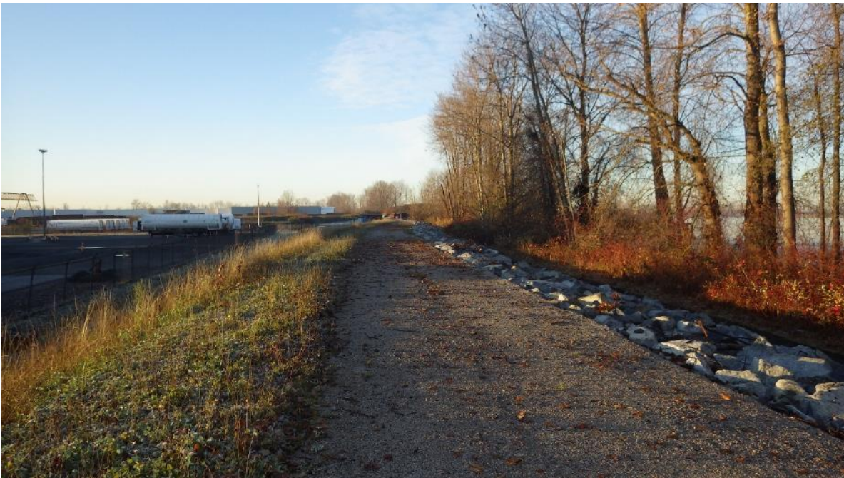
Photograph 8: View southwest along dyke, assessment area A. Assessment area C to the left. Note boulder armouring to the right, and trees that have likely grown within the last 50 years.
