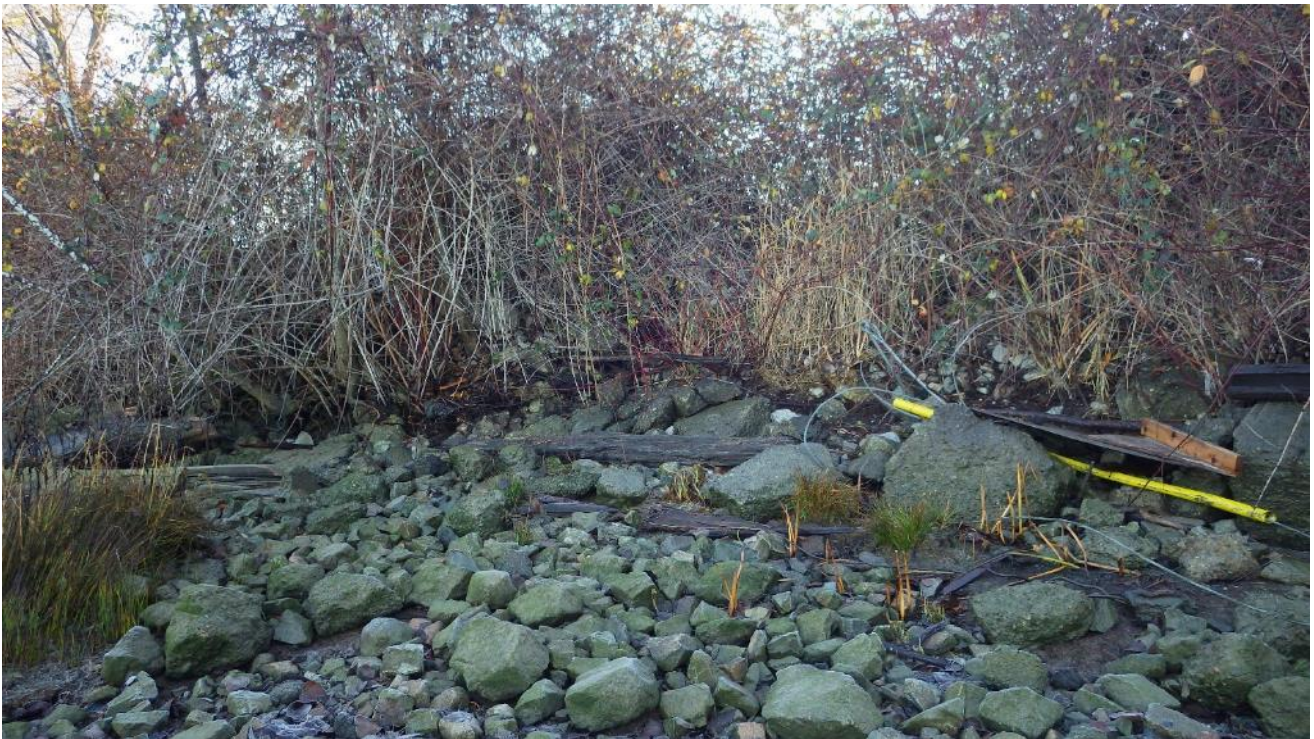
Photograph 12: View of rip-rap armouring from older dyke construction in assessment area A.
