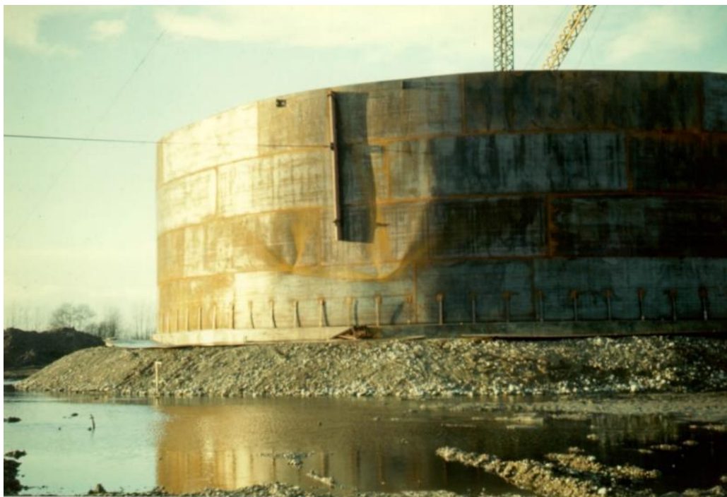
Photograph 2: Original storage tank under construction with original ground surface stripped, and gravel base over wooden piles (not visible) under the tank (image courtesy of FortisBC).
