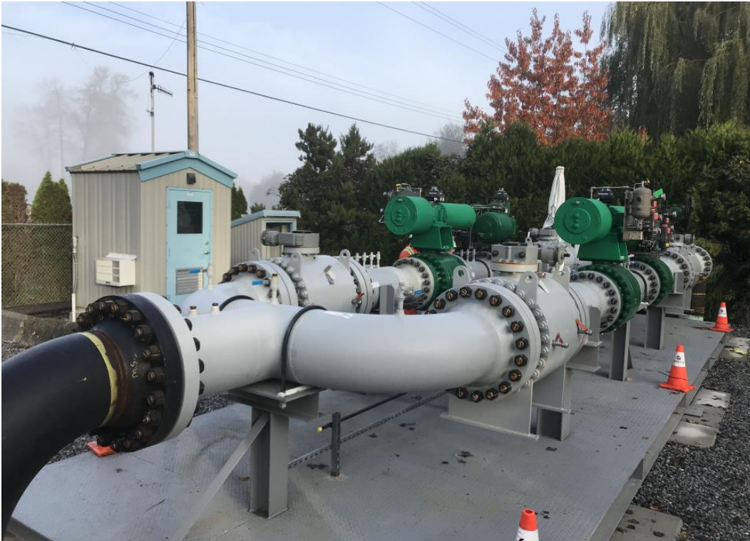
Figure 4-3: Example of Pressure Regulating Station
