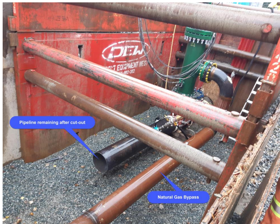
2 3 Figure 4-1(c): Example of a Pipeline Alteration with Natural Gas Bypass – Completed Alteration 4 and Bypass Removed
