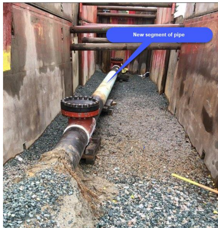
2 3 Figure 4-1(c): Example of a Pipeline Alteration with Natural Gas Bypass – Completed Alteration 4 and Bypass Removed
