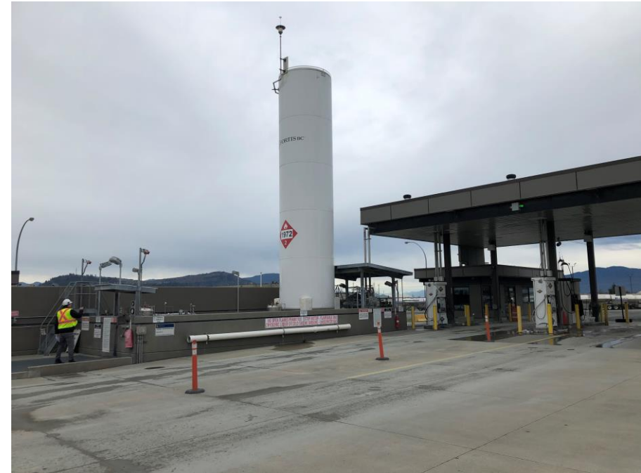
15,000 US gal vertical tank at Vedder Transport
