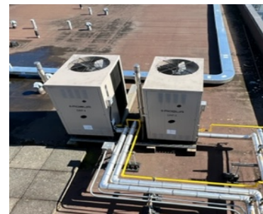
Installation of Outdoor Units on the Roof
