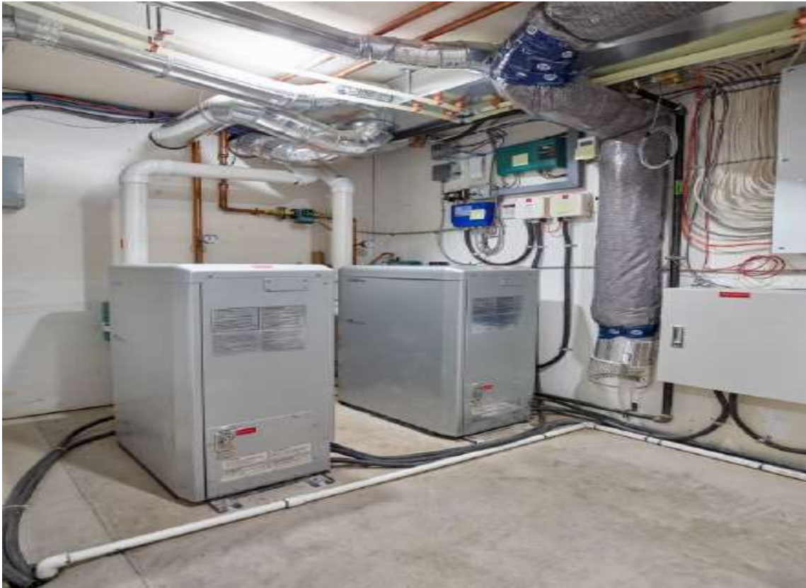
Figure 10-2: Installed Micro-CHP unit
