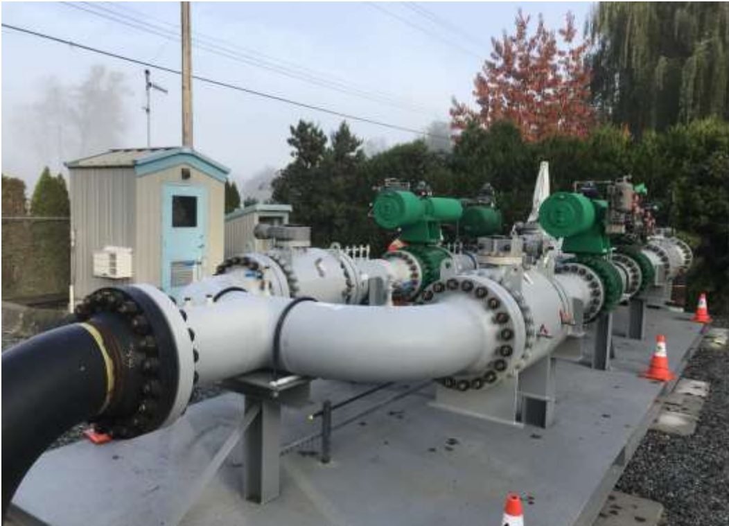
Figure 4-3: Example of a Pressure Regulating Station
