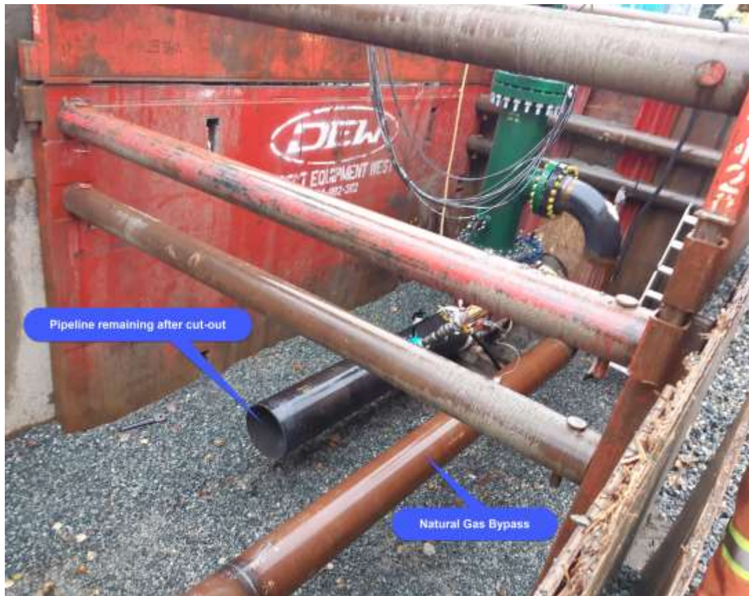
Figure 4-1(b): Example of a Pipeline Alteration with Natural Gas Bypass – After Cut Out
