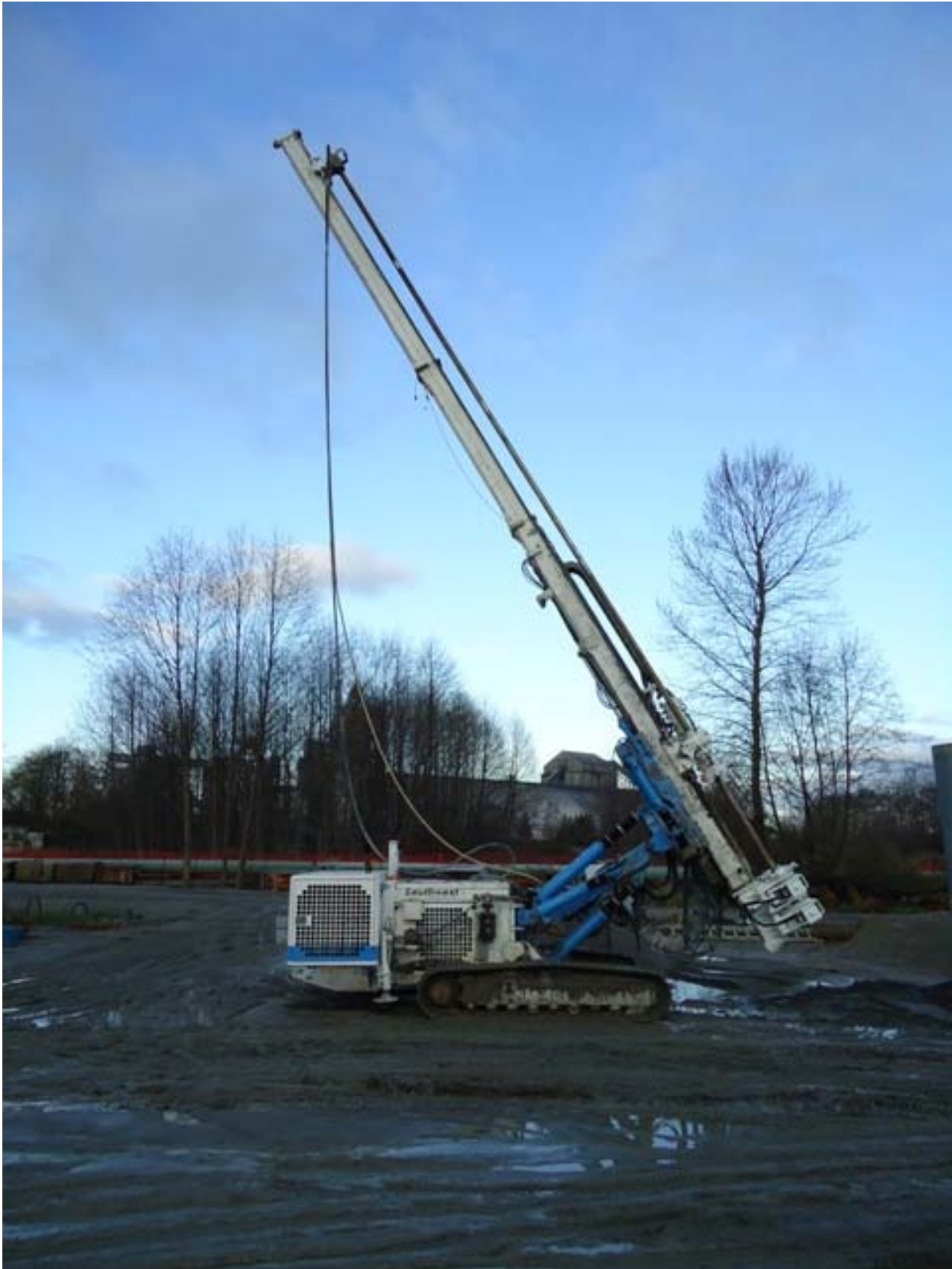
Mar 27, 2011 – Jet grouting rig
