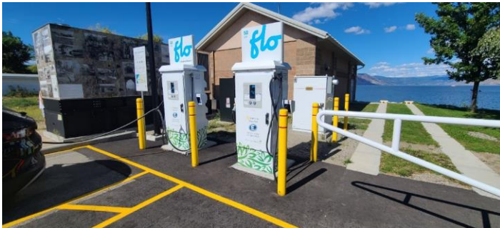
Figure 3-2: FBC's Naramata DCFC Site with Accessibility Considerations
