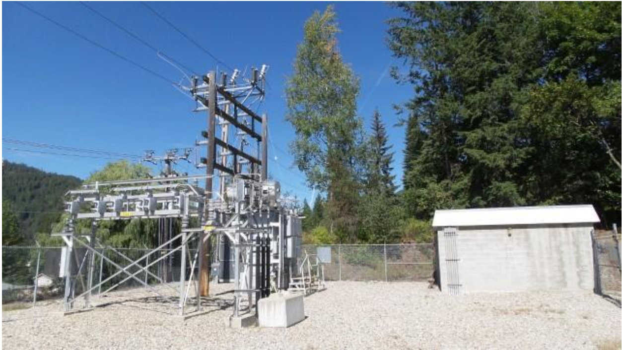
Figure 3-2: Existing Fruitvale Substation Ground Level View
