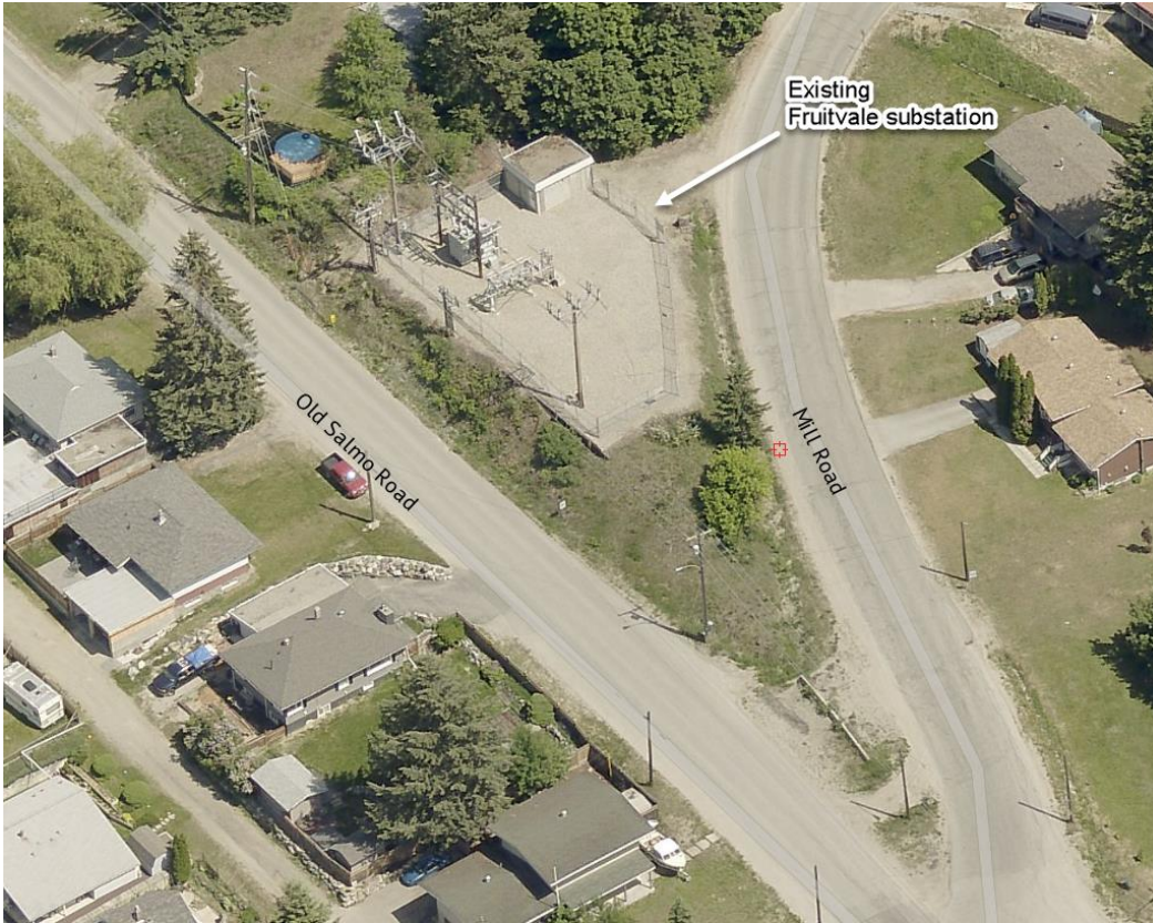
Figure 3-3: Existing Fruitvale Substation Aerial View
