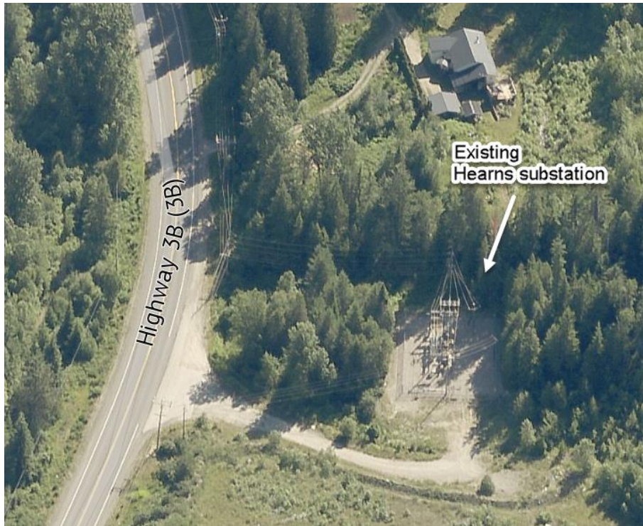
Figure 3-5: Existing Hearns Substation Aerial View
