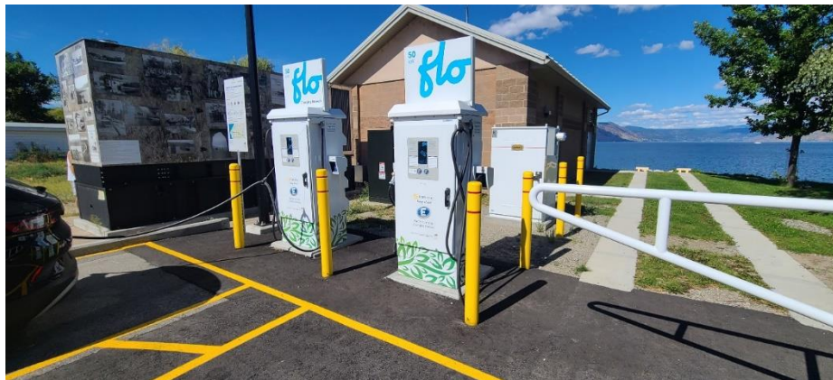
Figure 3-2: FBC’s Naramata DCFC Site with Accessibility Considerations
