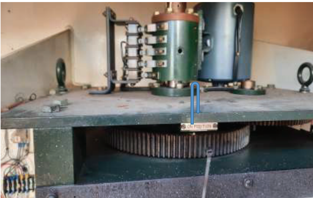
Figure 6 ASM T2 Misalignment of the gear mechanism
