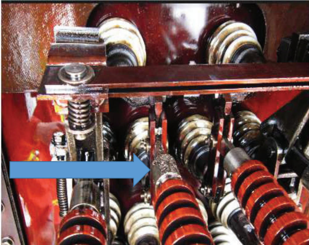
Figure 6 ASM T2 Misalignment of the gear mechanism
