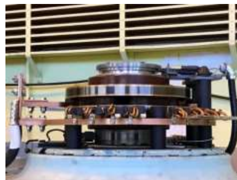
Figure B2-10: Exciter Brushes and Speed Sensor
