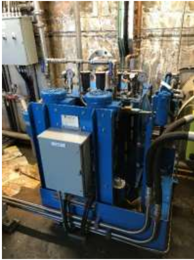
1 Figure B2-1: Bearing Oil Lubrication Unit
