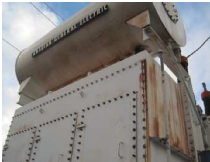
Figure 3: Tap changer compartment and conservator showing surface corrosion
