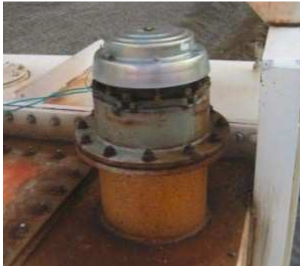
Figure 1: Main tank pressure relief device, the debris below the device is evidence of an oil leak
