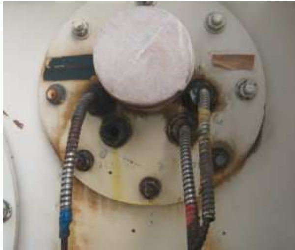
Figure 2: Signs of an oil leak on the side of transformer tank are visible stemming from the thermal
