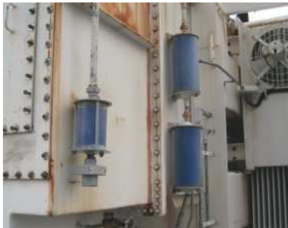
Figure 5: Desiccant columns shown with new desiccant installed
